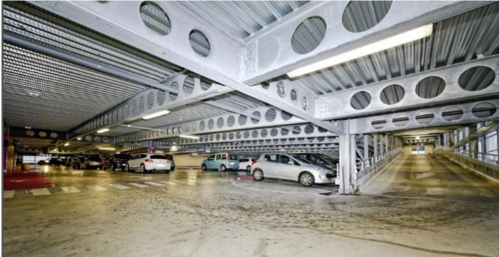
Figure 1. Parking structure (Arcelormittal, 2020a)
