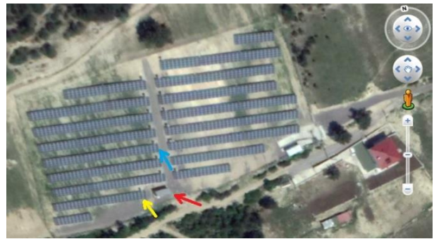
Figure 1. Satellite image of the pv power plant. Transformer building (red arrow), shaded string (yellow arrow) unshaded string (blue arrow).
