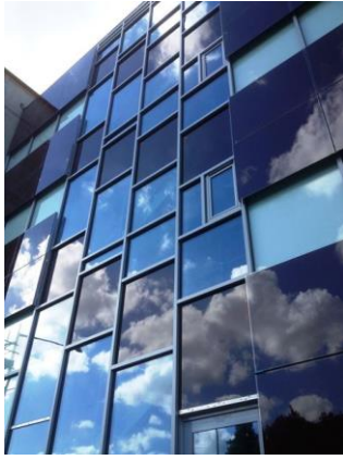
Figure 6. Polysolar (PS)-A opaque series panels, Future Business Center, Cambridge shelters [4]
