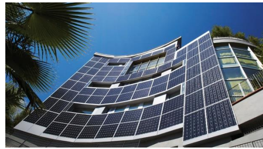
Figure 19. (a) Solar panel BIPV façades glass curtain wall with solar modules cell cladding and (b) an example of its application [33]
