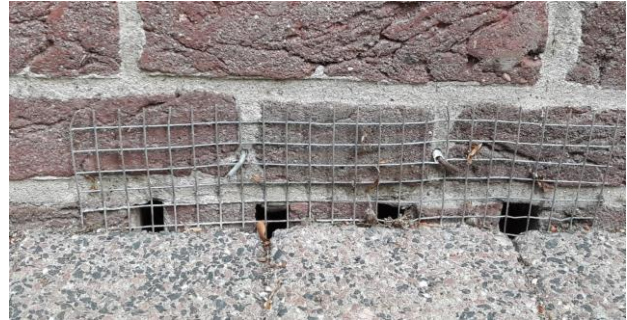
Figure 1. Entrances to the wall cavity at ground level.
