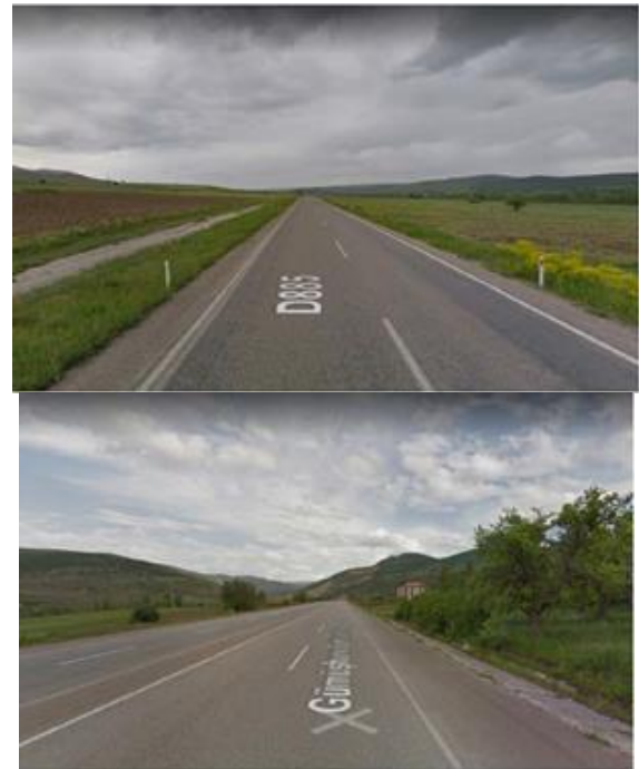
Figure 4. Open Road-1 (OR1- two lanes) and Open Road-2 (OR2-four lanes)
