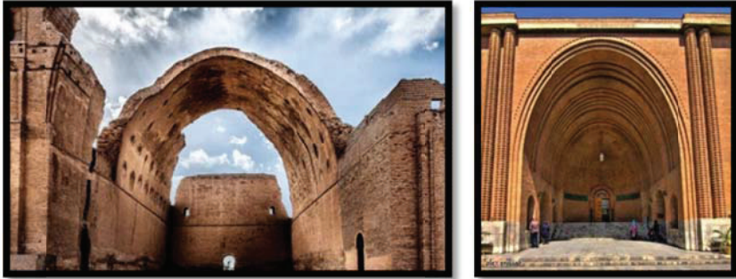
Figure 5: Left to right: the historic Sassanian Ctesiphon Vault, the entrance of the National Museum of Iran 3233
