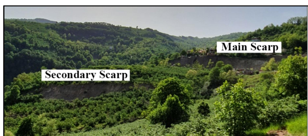
Figure 9: General view of Sağlık District landslide from the northwest, which has a two-part structure.
