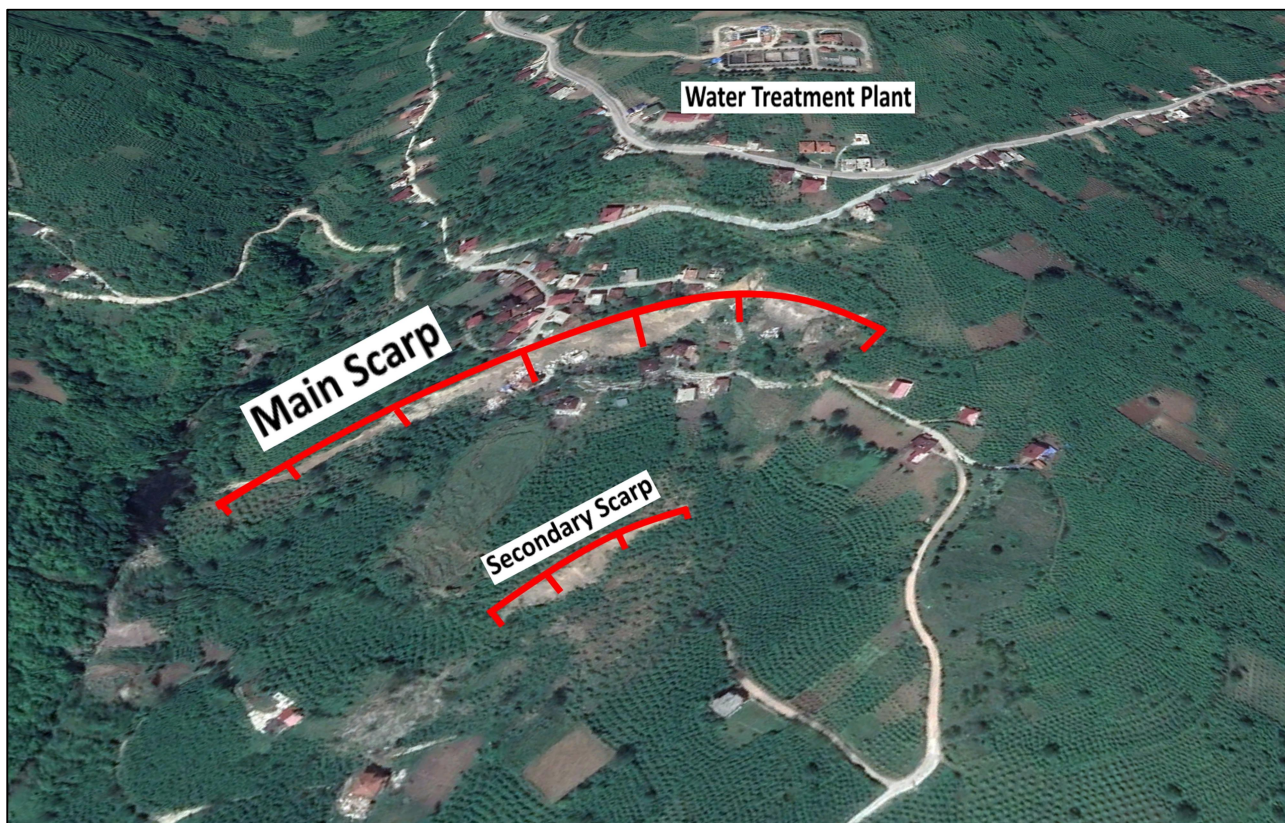
Figure 8: The landslide area and its surroundings.
