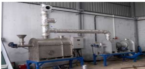
Figure 1. Settlement of the dryer and pyrolysis unit.
