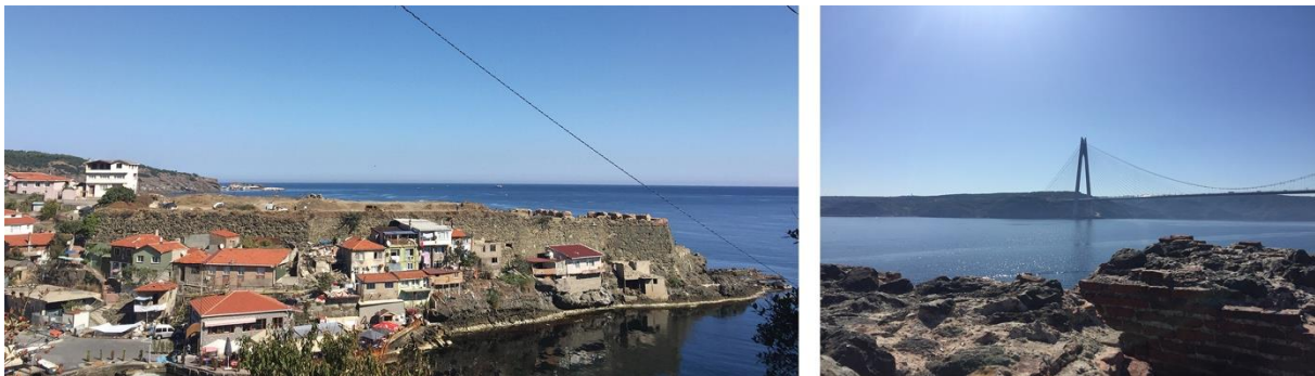
Figure 3. Garipce Castell and The Third Bridge (Source: Authors).
