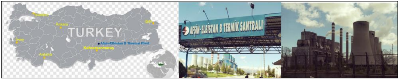
Figure 1. Geographic location of Afşin-Elbistan B thermal power plant
