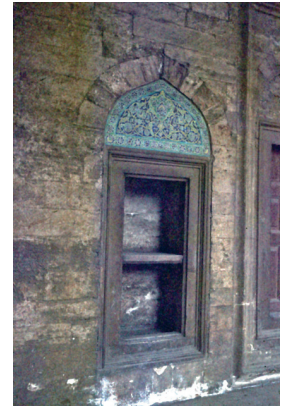
Figure 15: Cuerda seca window lunettes of the Kara Ahmed Pasha Mosque, courtyard view, 1986. SALT Research, Kemali Söylemezoğlu Archive, TSOH100002.
