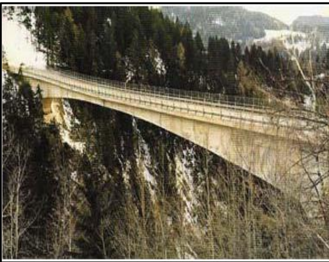
Figure 1. Historical buildings produced with lightweight concrete: The bridge in Italy (El Zareef, 2010).
