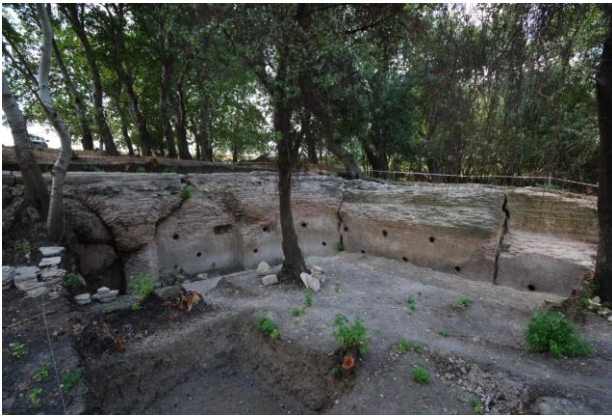
Fig.7. Body walls with oval corners in the cistern and offsets and damage identification relief studies of walls due to probable large earthquake.
