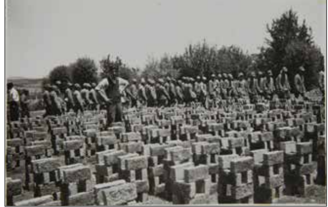
Figure 16: Brick drying process at an institute (IHTBV). / Enstitüde tuğla kurutma aşaması (IHTBV)
