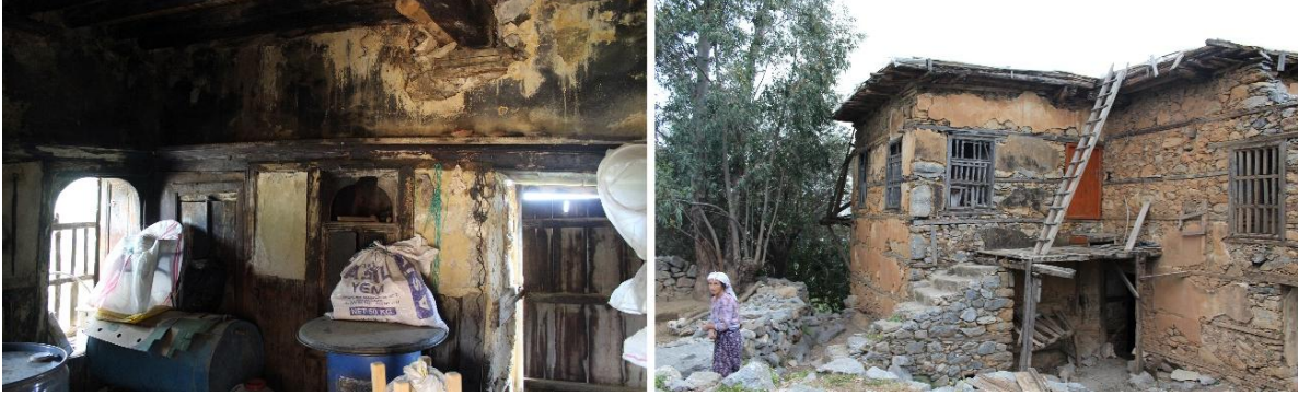
Figure 17. Building Interior Detail and Building Entrance
