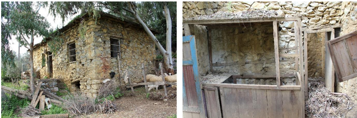
Figure 6. South East View
