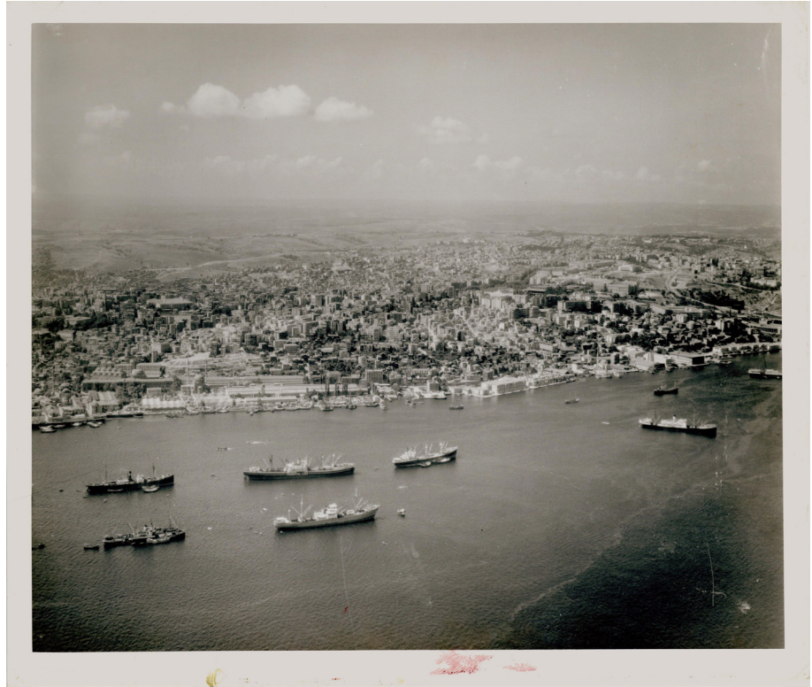
Figure 14: Aerial photograph of the Port of Galata and the landing ships, 1950. SALT, AHISTBEYO095.
