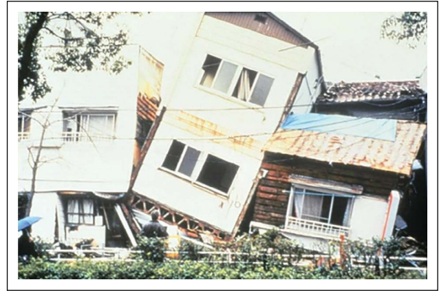
Figure 3. Wooden structure damaged in the Great Hanshin earthquake [9].
