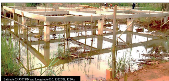
Photo 2: Raised foundation on wetlands at Mulang (Field Survey, 2020).
