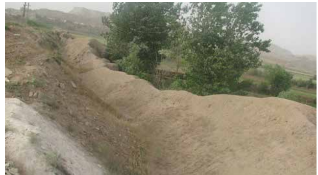
Figure 7: Rampart and Fence of Rabaz alongside Imam Ali Highway (authors). / İmam Ali Yolu yanındaki Rabaz suru.
