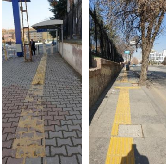
Figure 4. Accessible Routes (Photograph: Gamze MIZRAK, February 2021)
