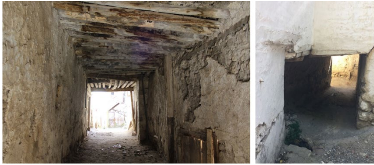
Figure 16. Susaklı Neighborhood Covering II (Photo:Author)
