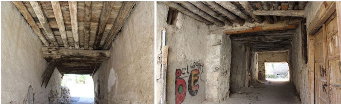
Figure 11. Coverings Constructions (Photo:Author)
