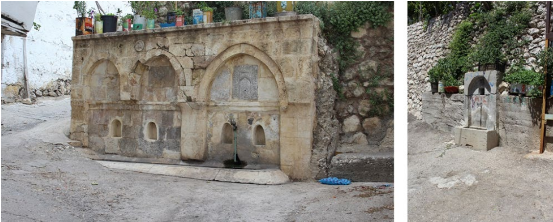
Figure 8. Street Fountains (Photo:Author)
