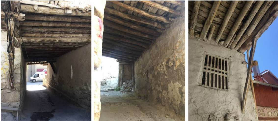
Figure 12. Wooden Beams (Photo:Author)
