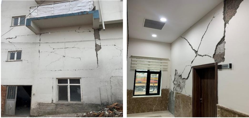
Figure 11 In-plane damage
