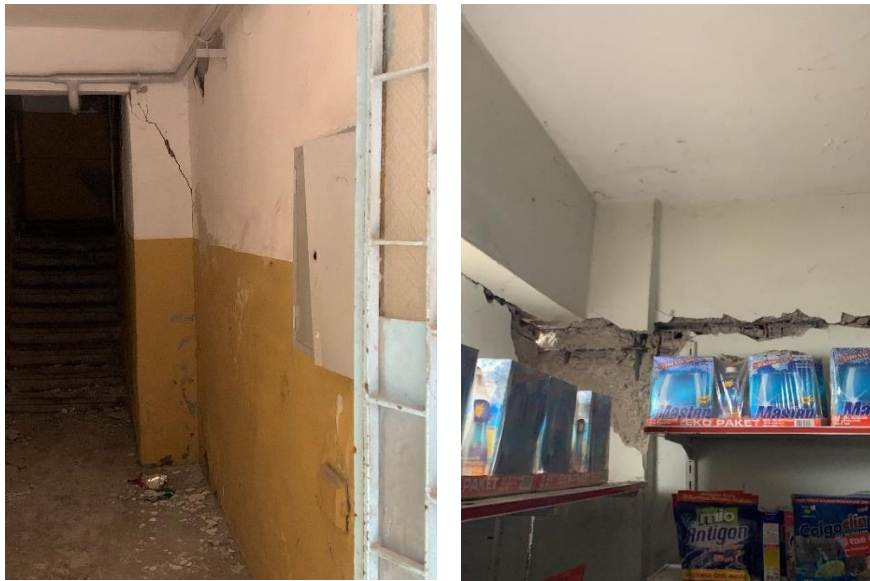
Figure 10 Strong beam–weak column
