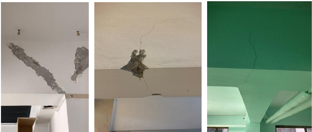
Figure 9 Beam damages
