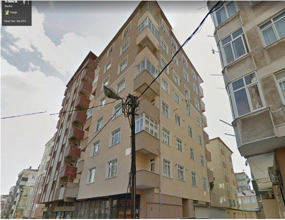
Figure 8. Yeşilyurt Apartments Before Collapse
