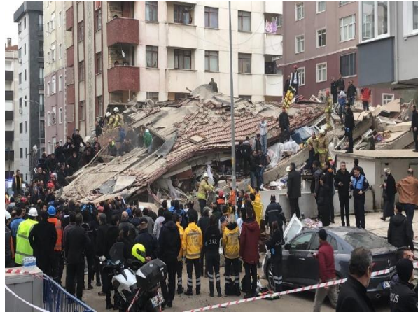
Figure 9. Yeşilyurt Apartments After Collapse
