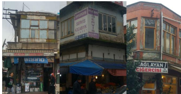
Figure 7. Facades from Unkaparı shops, 2019, January 11.
