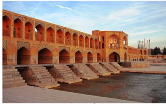
Figure 10. Khaju Bridge, Isfahan, Iran
