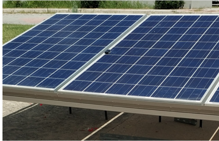
Figure 1. Photovoltaic System Installation
