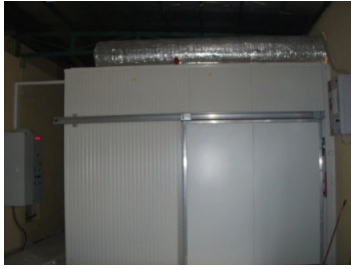
(a) general view of cold storage
