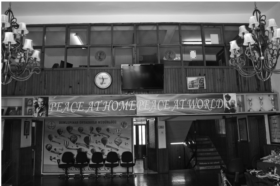
FIG. 10 Middle floor added in mid-1970s (by author).
