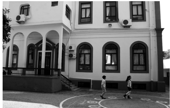
FIG. 6 Subsidiary structure at the northern façade (by author).
