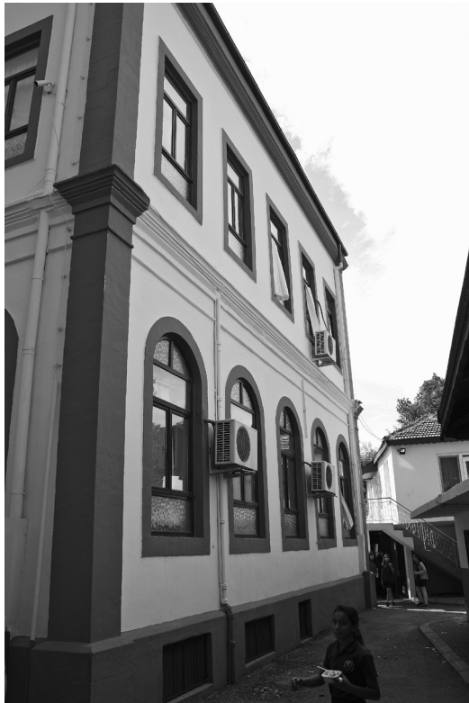
FIG. 8 Western façade (by author).
