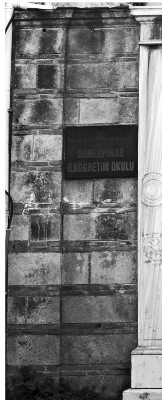
FIG. 16 Masonry technique at either sides of the gate (by author).
