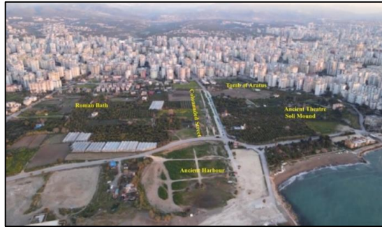
Figure 21. Soli-Pompeipolis under the pressure of urban development
