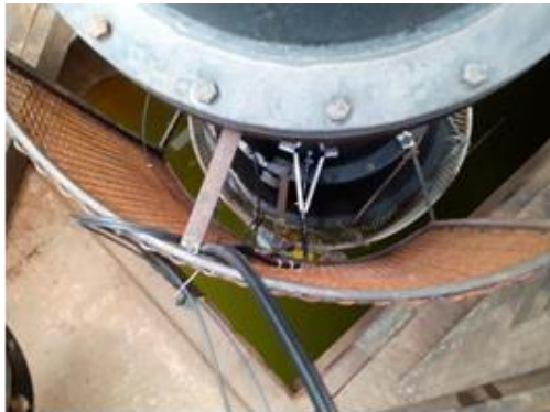
Figure 9a. Placing the pump to the test bed
