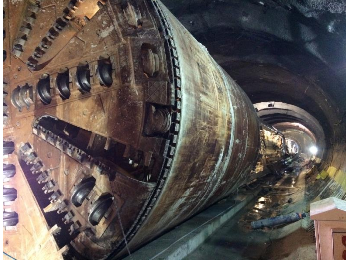
Figure 11. EPB-TBMs in the M5 Metro Tunnel
