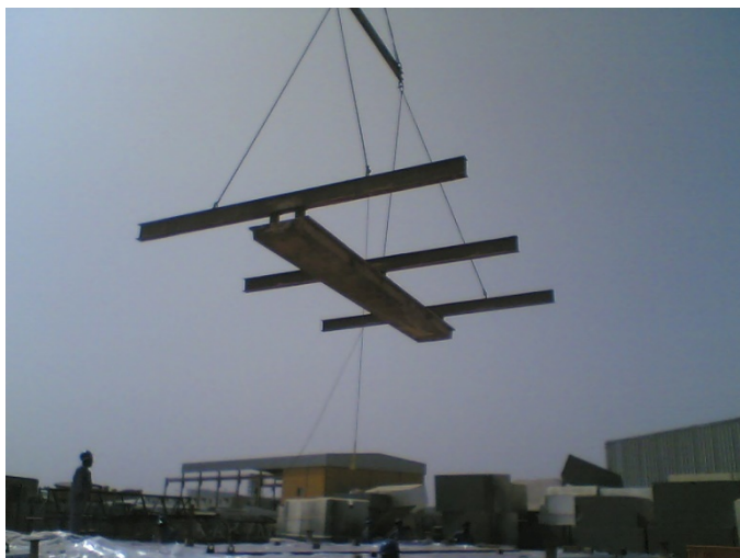
Figure 4. Service duct lifting
