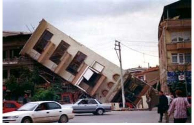
Şekil 6. Devrilen bina No:4 (H=15,00 m, B=5,00 m), (H/B=3,00) [24] (Overturned building No:4 (H=15,00 m, B=5,00 m), (H/B=3,00) [24])
