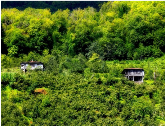
Photograph 2. Wooden architecture in Machakheli (Balci, 2021: 11).
