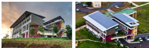
Figure 1. General view of ENERPOS (left) and aerial view (right) with the PV roofs. ENERPOS is composed of two parallel wings separated by a green patio. A car park is located underneath the patio and the left wing.
