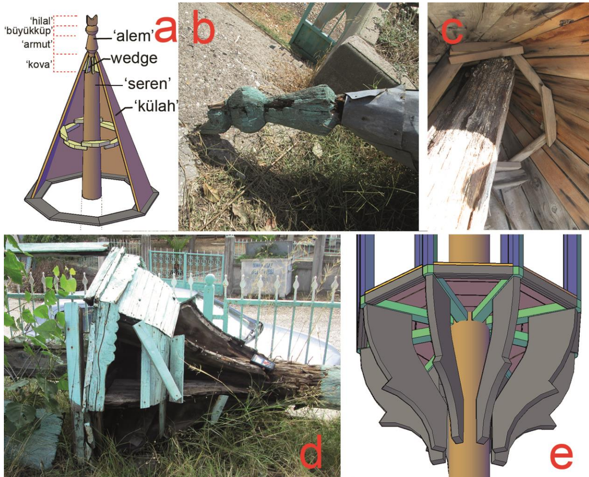
Figure 9. 3D model (a,e) and photographs of Yaylaalan old mosque minaret taken in 2015 (b,c,d)
