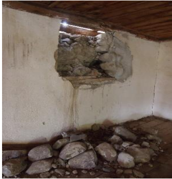
Figure 22-23. Deteriorations on stones
