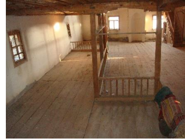
Figure 6. Southeast wall of the main prayer area
