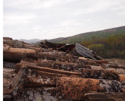
Figure 24. Deterioration on the roof
