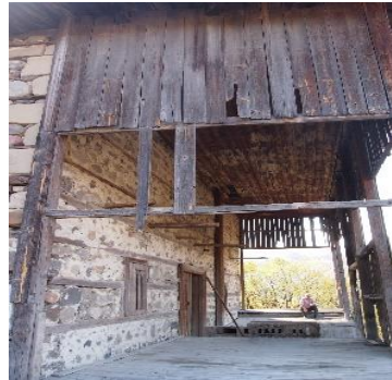
Figure 25-26-27. Deterioration on timber parts
