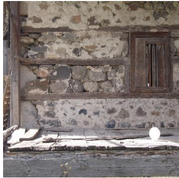
Figure 22-23. Deteriorations on stones
