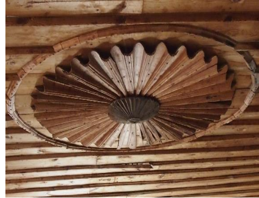
Figure 18. Center covering of the ceiling
