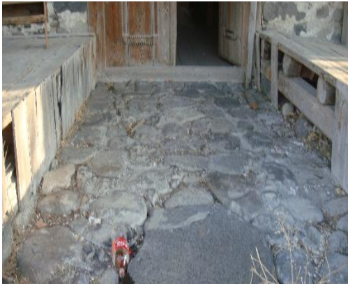
Figure 19. Latecomers' portico floor
