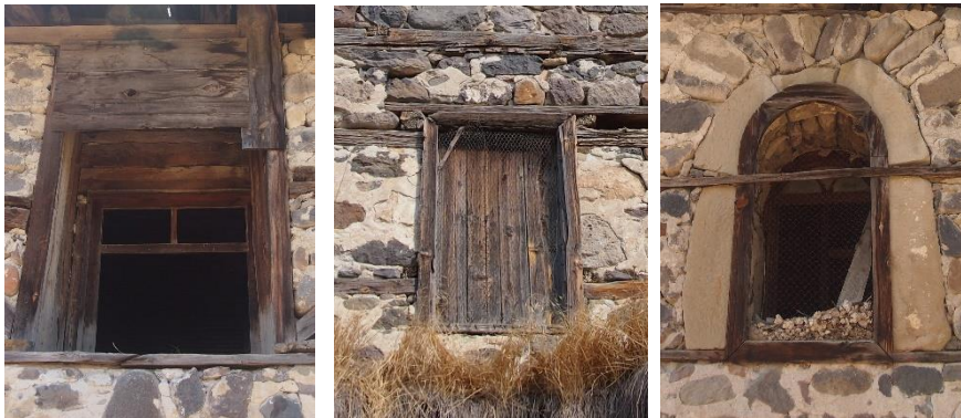
Figure11-12-13. Windows of the main prayer area
