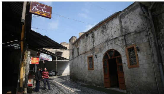
Figure 15. Abamor Ice Factory after Restoration (Betül BEYAZ HKU Department of Interior Architecture Graduate Student)
