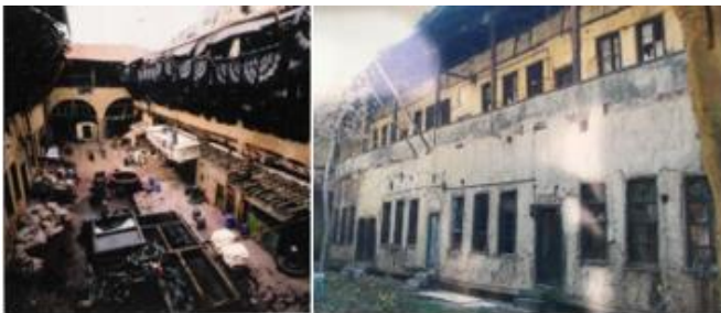
Fig. 13. Yazmacılar Han courtyard view (Before Restoration) [15].
