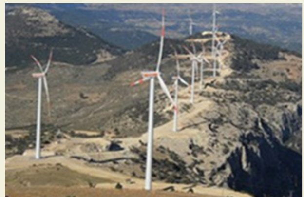
Fig. 11 Wind power plant of Mersin province
