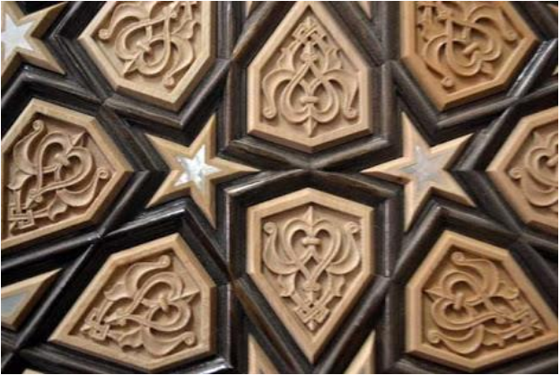
Figure 9. The general view of the geometric blocks, narlama and keel bars.
