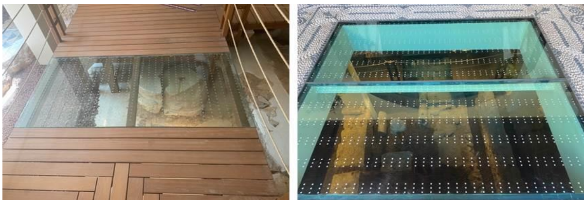
Figure 16. Screen Printing With White Dots on Laminated Glass Flooring (Original, 2021)
