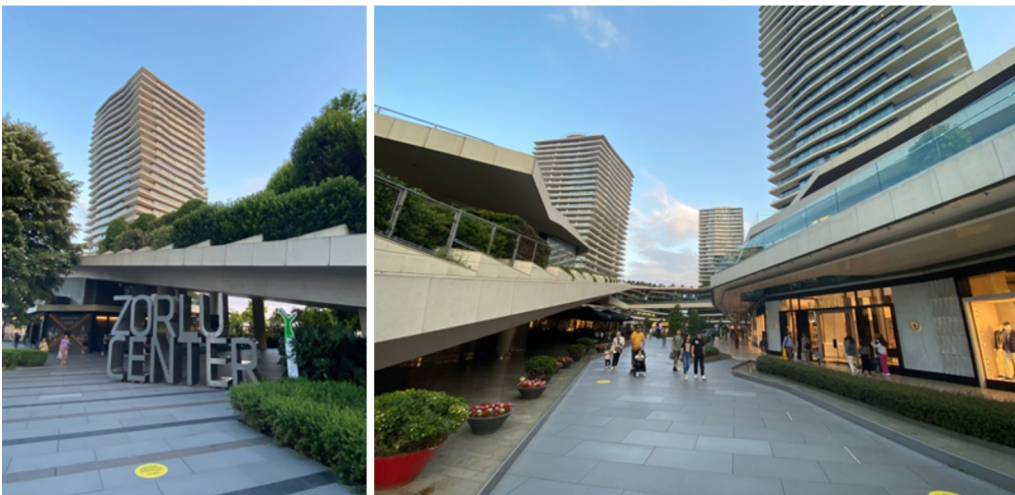
Figure 6-7. Zorlu Center tower, shell formation and courtyard/centre/square (Authors Archive, 2021).
