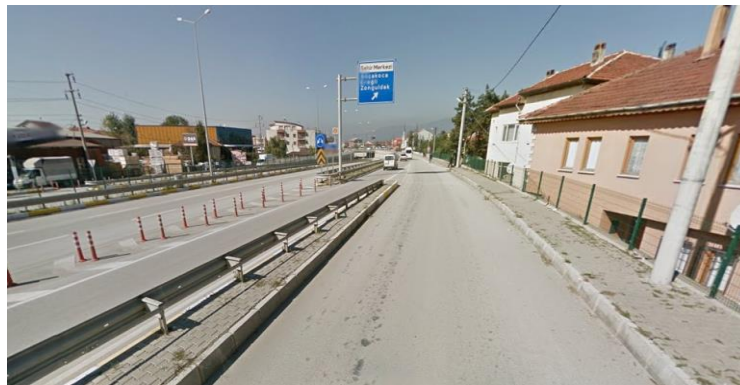
Figure 5. Side road connection.
