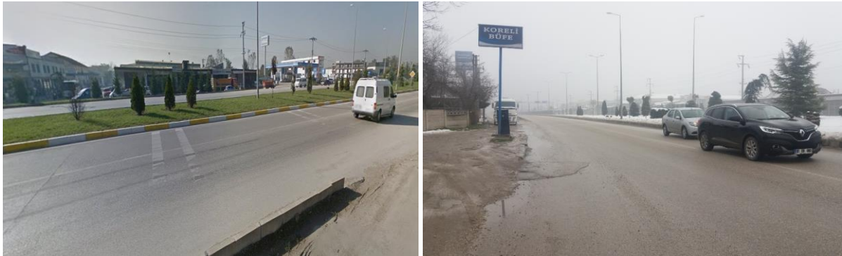
Figure 8. a) Section with side road connection, b) the section where the highway narrows after the side road connection.
