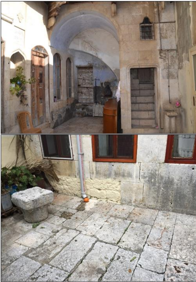
Figure 13. With respect to the comparative study on the trace on the wall and the one on the adjacent building lot no: 2060, and the statement of the inhabitant in the adjacent building in the current situation, the presence of a platform can be proposed.
