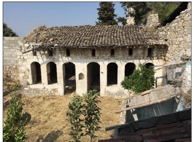
Figure 12. Façade configuration of the building on the plot no: 2054
