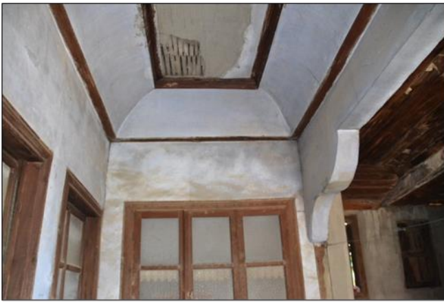
Figure 7. The curvilinear support that forms the border between the windows in the sofa and the decorated timber ceiling of this area and the covering under eaves that was added in the later periods
