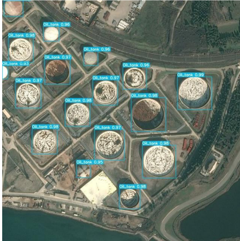
Fig. 6. Partly visible oil tank examples (top left).
