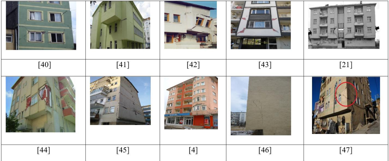
Figure 5. Damages observed in heavy overhangs after different earthquakes in Türkiye
