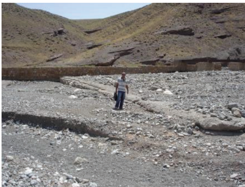
Figure 12 - View from the crest of the underground dam in Sufi River (Photo by B Vaheddoost).
