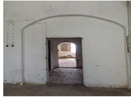
Figure 9. The stone wall, which was built later, that provides the transition to 1-03 office room on the northeast facade wall of 1-01 Entrance-Hall
