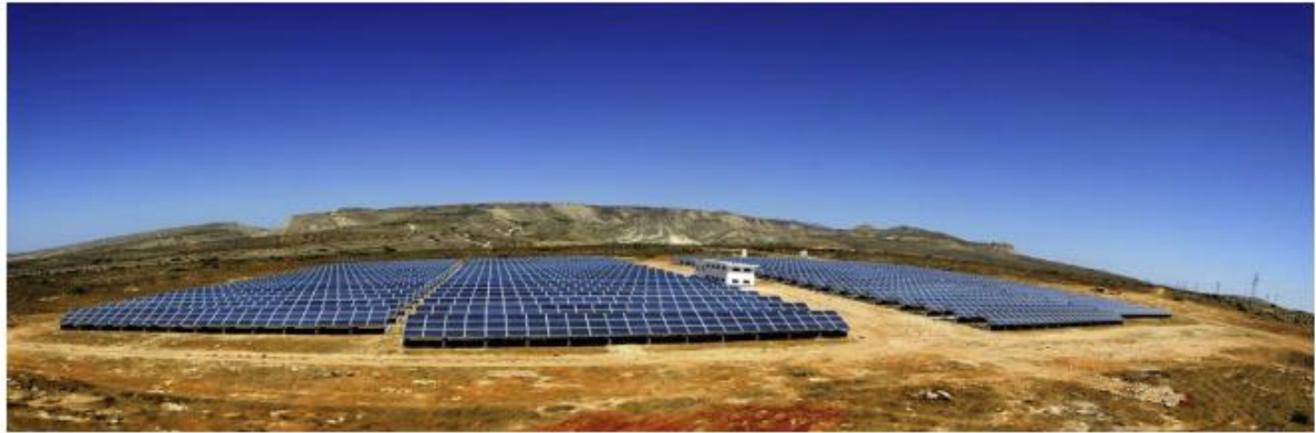
Figure 1. Site view of Serhatköy PV Plant (Maltini and Minder, 2015)
